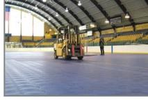
ED Ice can handle weight loads up to 20,000 lbs. per square foot (static load).
