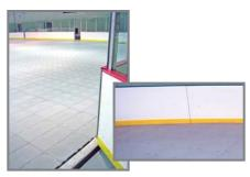
Tiles can be cut with a circular saw to fit snugly against dasher boards.
