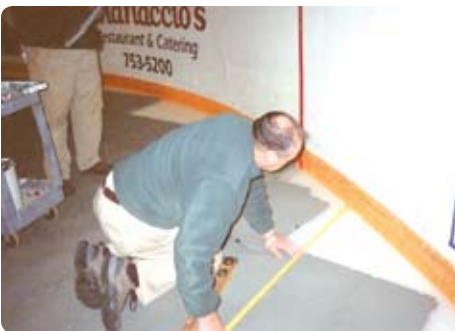
Radiuses can be cut with a jig saw for a perfect fit.
